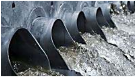
Scottish sewers 'could warm Glasgow through winter'
